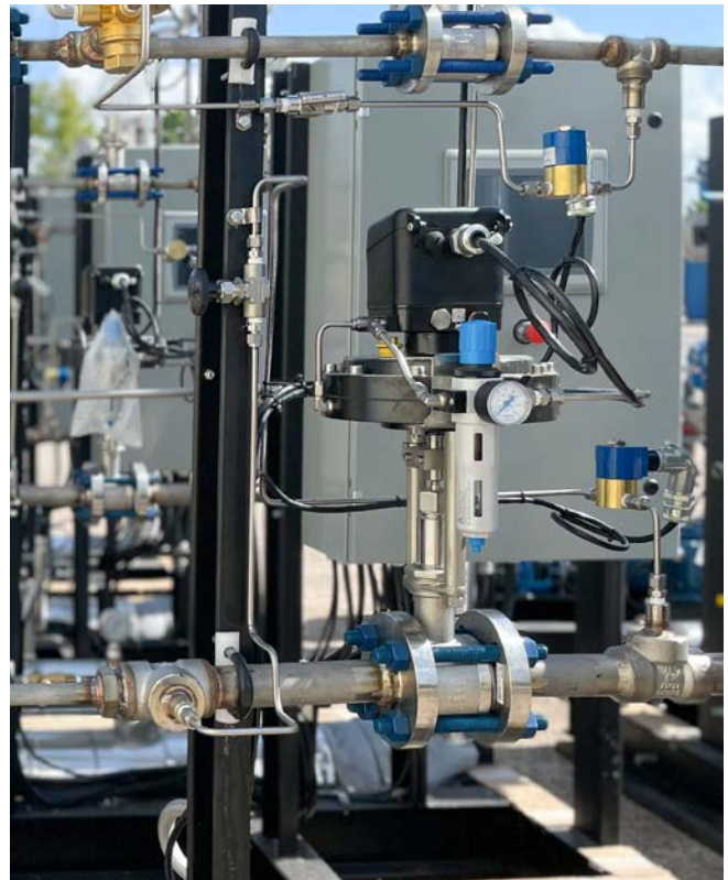
Figure 02: Due to the high rangeability of the sliding gate valve, the Thermal Well Generator now requires only one valve for gas and one for air.
