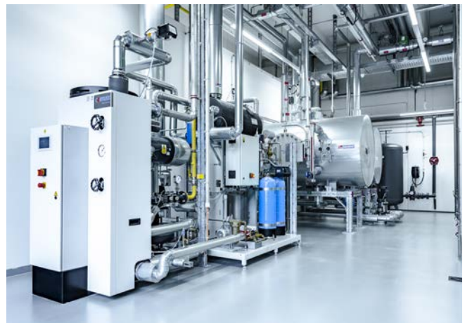
A Junior 400 TC fast steam generator from CERTUSS feeds the steam test bench in the power station at Schubert & Salzer.
